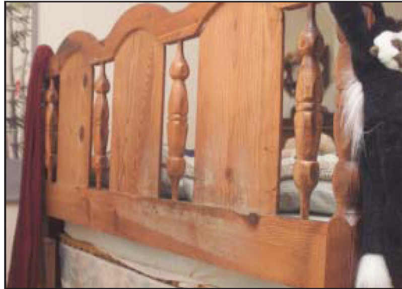
Mold growing on a wooden headboard in a room with high humidity.
