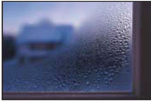
Condensation on the inside of a windowpane.
